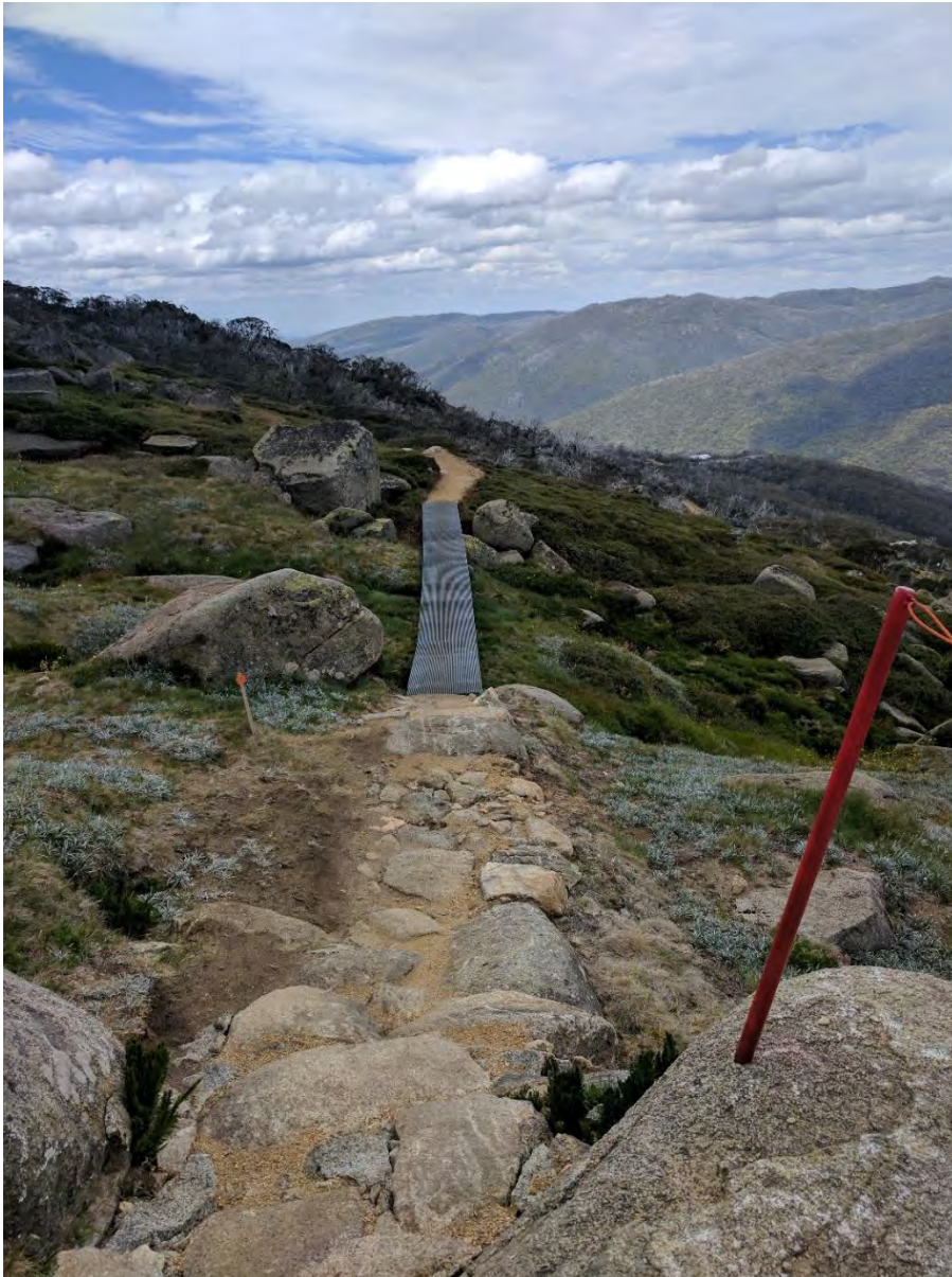
Figure 34: Example of rock armouring on the All-Mountain Trail
