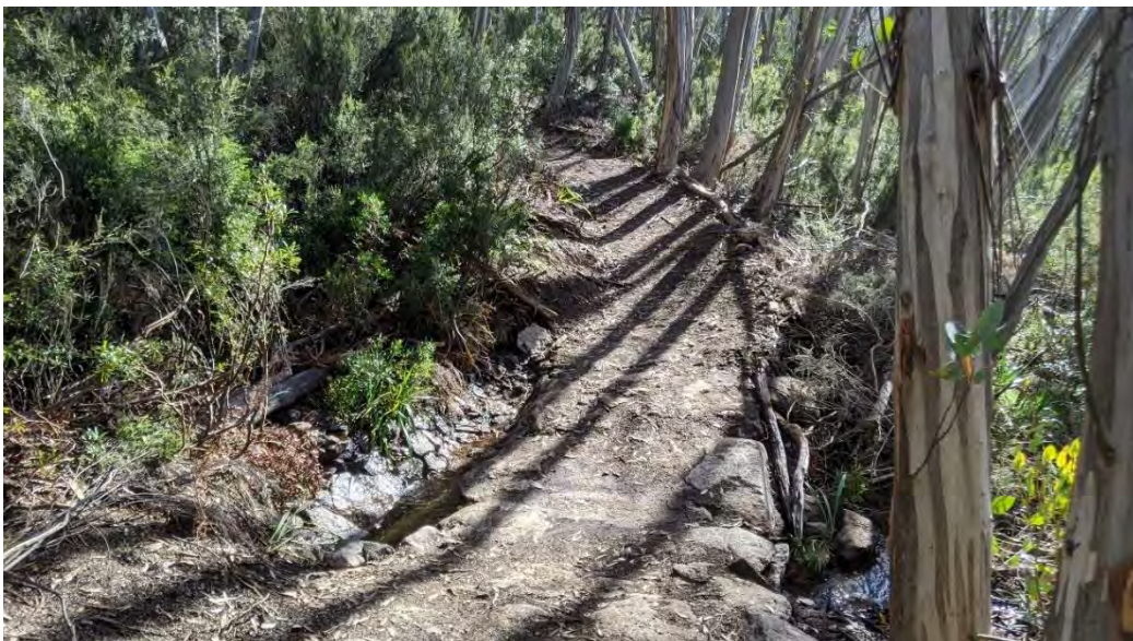
Figure 33: Example of rock armouring on the Lower N4 Trail
