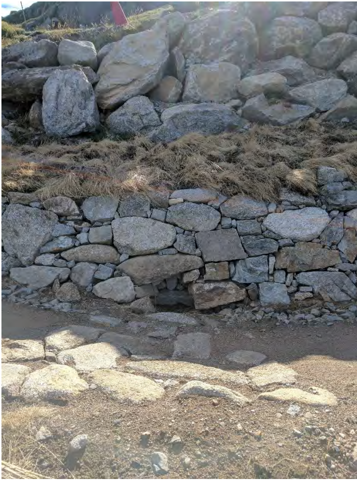
Figure 32: Example of a drain dip, rock hardened on the All-Mountain Trail
